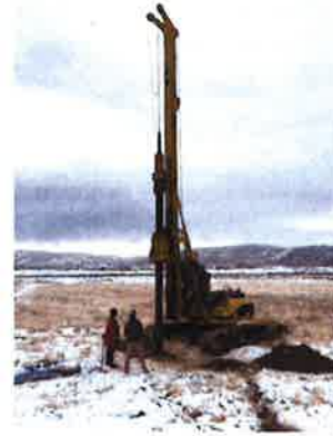
Groundwater Investigation Cold Springs Water Reclamation Facility
